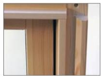
To make sure the frame is set properly, check the gaps at the closure of the sash. If the vertical gaps are parallel with the gap at the bottom in a slightly opened position, then the frame is correctly aligned, and the top brackets can be fixed.
