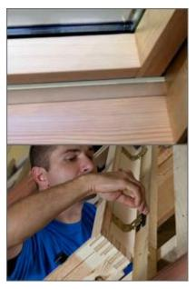
A plastic wedge is supplied to pack the bracket where there is an uneven rafter.
